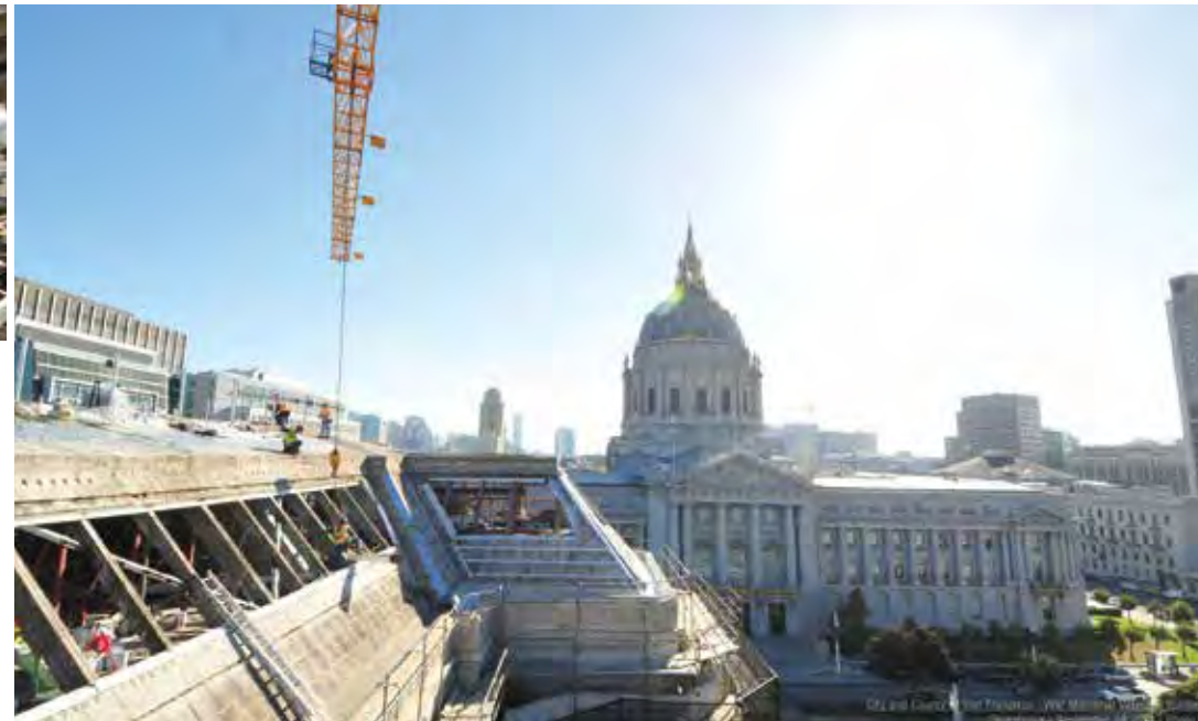
Originally completed in 1932, the War Memorial Veterans Building was where President Harry S. Truman and other heads of state signed the United Nations Charter in 1945. Through OneSF, this historic resource underwent a seismic retrofit, systems were upgraded to be more energy-efficient, and safety features like sprinkler and fire alarm systems were added.
