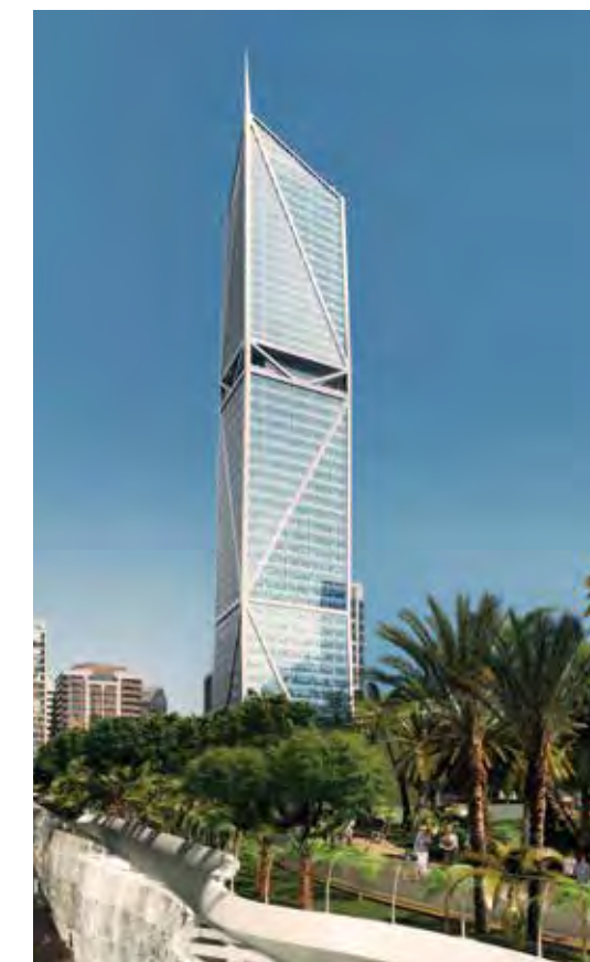
The 181 Fremont Tower was designed to significantly exceed code standards and is expected to be reoccupiable directly after a large earthquake.
